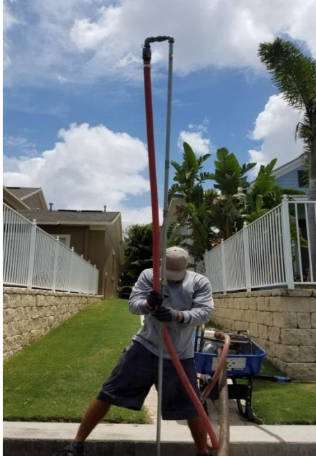
Photo No. 4 – Advance of probe by hydraulic jetting.
