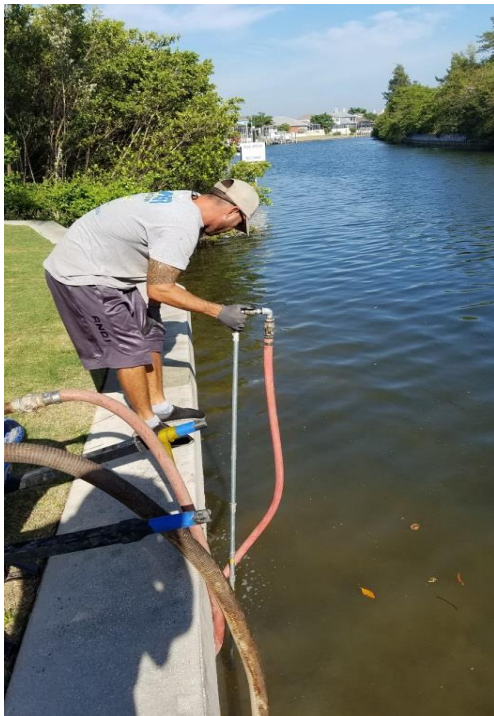
Photo No. 6 – Probe advanced at incline under sheet pile.
