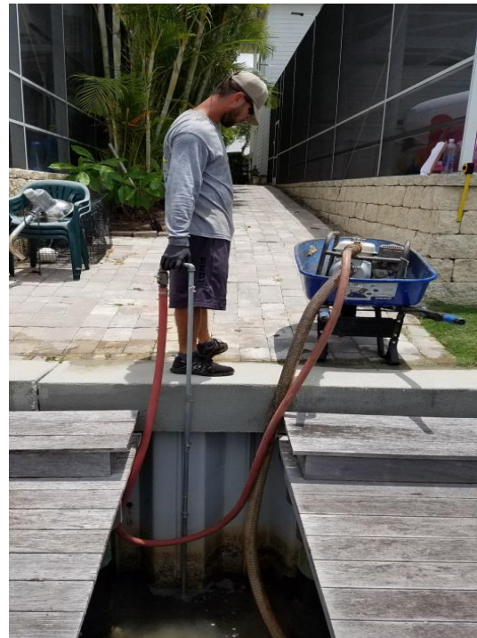
Photo No. 7 – Probe retrieved from under sheet pile to infer embedded sheet pile tip.
