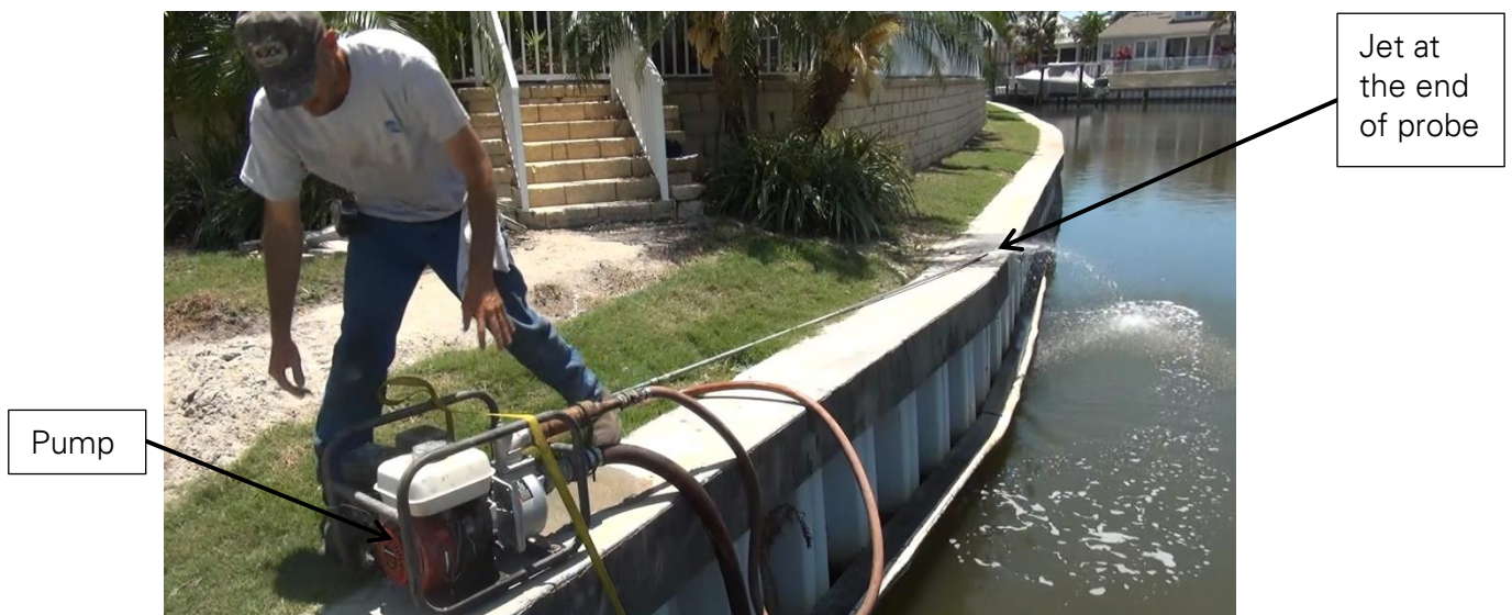
Photo No. 3 – Hydraulic Jetting Assembly
